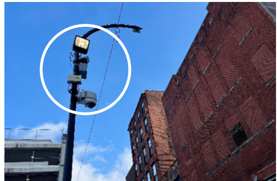
Figure 2: Rochester Police Department Blue Light Camera on Division Street
